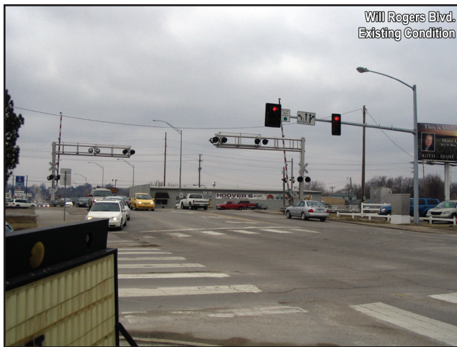
Figure 6: Existing Condition at Will Rogers Boulevard with At-Grade Public Railroad Crossing
