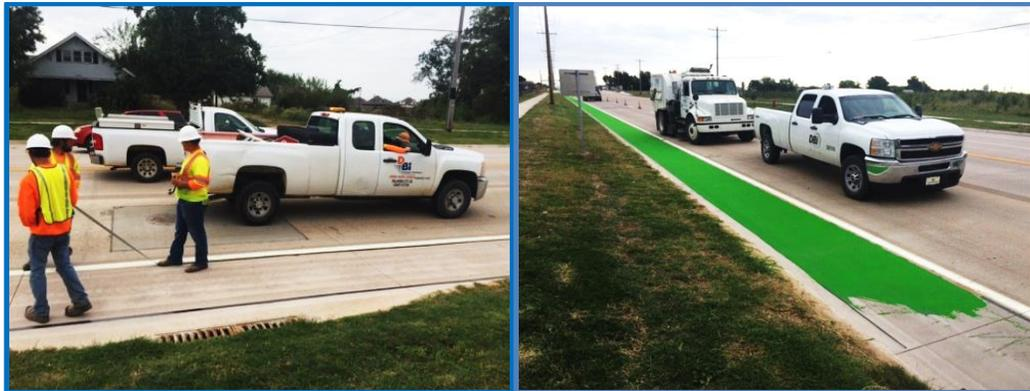
Figure 2. Road crew installing green bike lanes on Cedar Lane in Norman, Oklahoma
