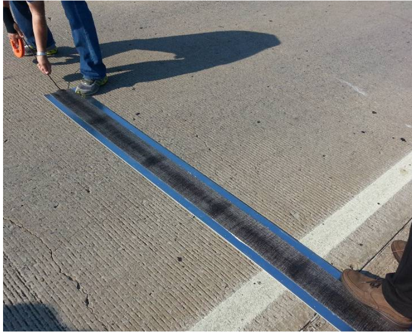
Figure 3.4 Pocket tape insertion using fishing wire and lubricant
