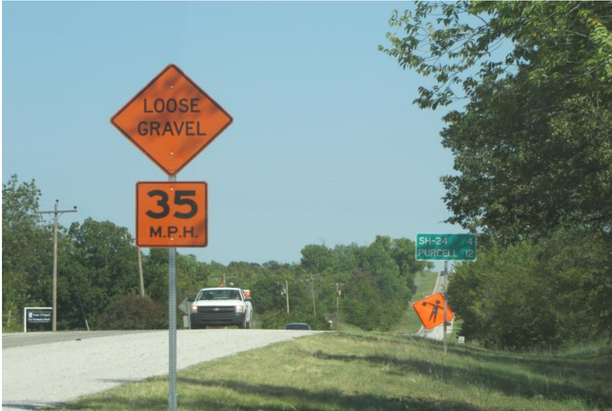
Figure 6.9 Traffic Control Signage and Pilot Car for Test Section Installation
