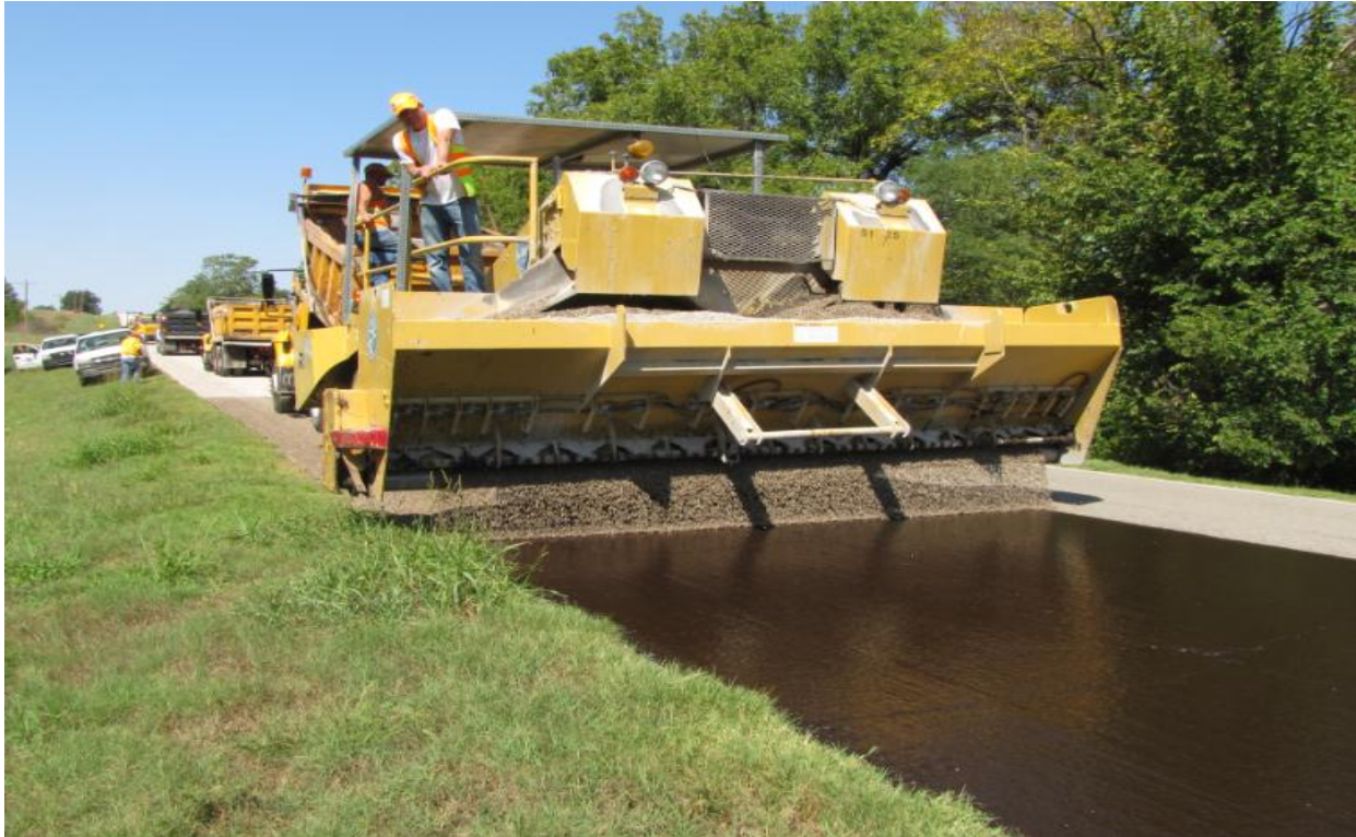
Figure 2.1 Chip Seal Installation
