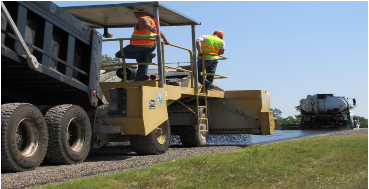
Figure 6.6 Chip Seal Construction: Distributor, Chip Spreader and Dump Truck
