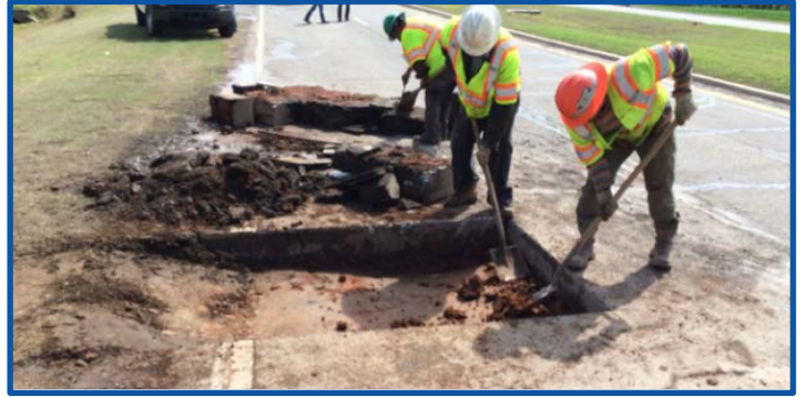
Figure 8. Test Pit to obtain Bulk sample from Layer 3
