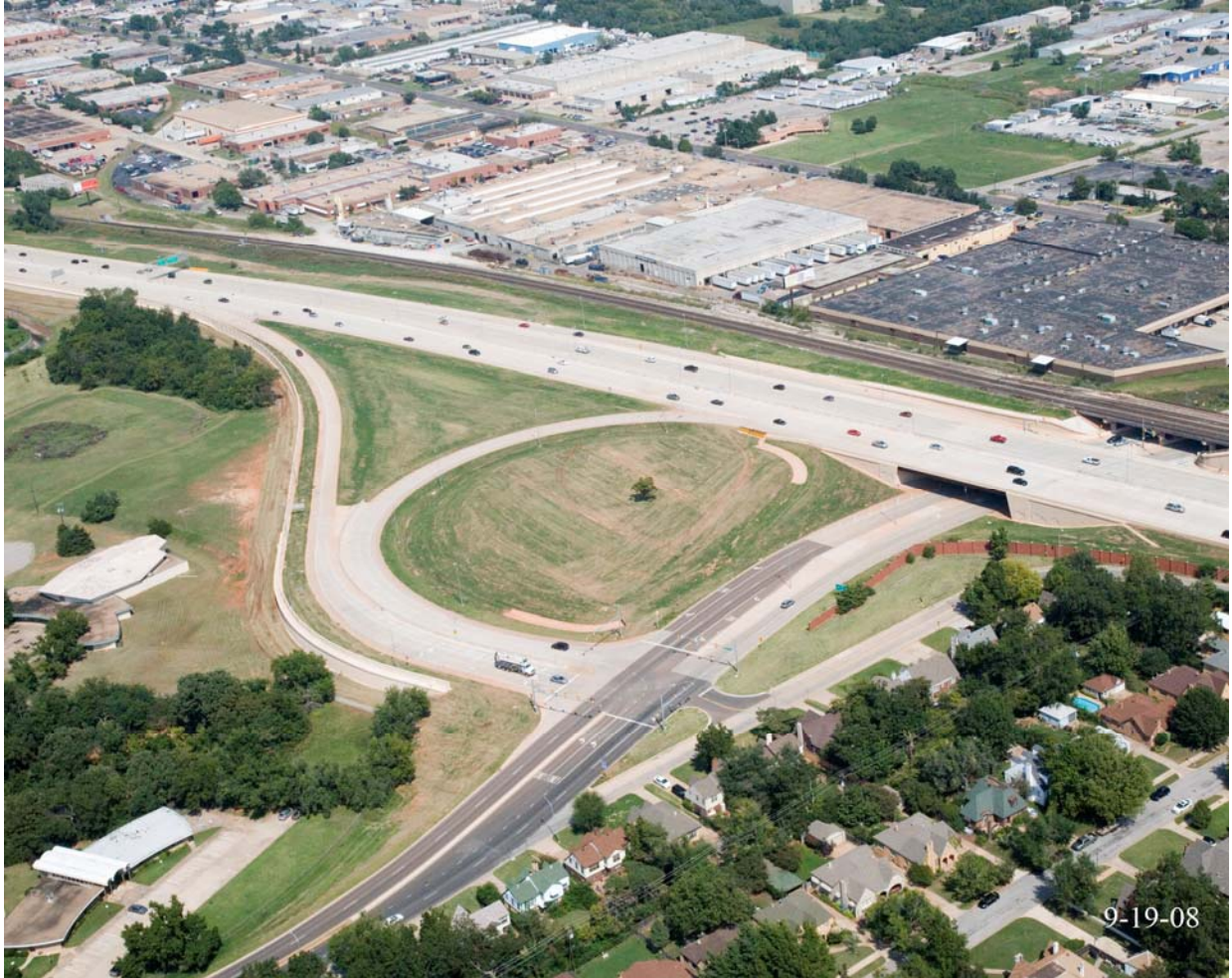
The I-235 at N.W. 36 th St. Interchange project in Oklahoma City, completed in September 2008, was honored with the regional America's Transportation Award Monday. The award recognized ODOT and its partners for the top-tier construction, early completion, saving of taxpayer money and adding innovative public art on the $27 million project northwest of the state Capitol.
