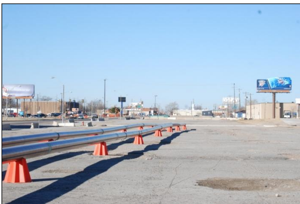
Viewpoint 10: Former I-40 right-of-way at Shields Boulevard, looking west
