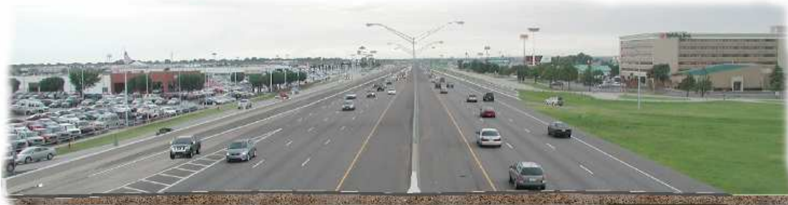
ROBINSON STREET TO MAIN STREET LOOKING SOUTH
