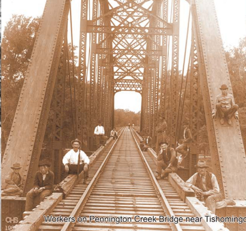
Workers on Pennington Creek Bridge near Tishomingo
