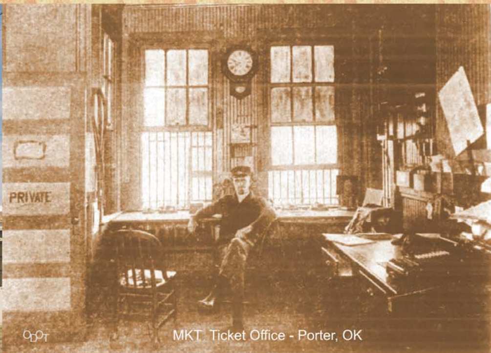
MKT Ticket Office - Porter, OK
