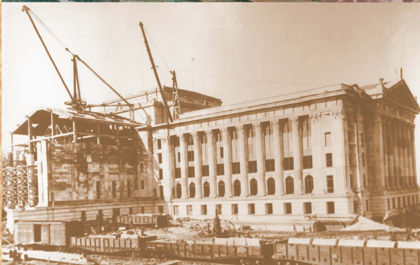
Cars with stonework along rail spur built during the construction of the State Capitol 1915-1916
