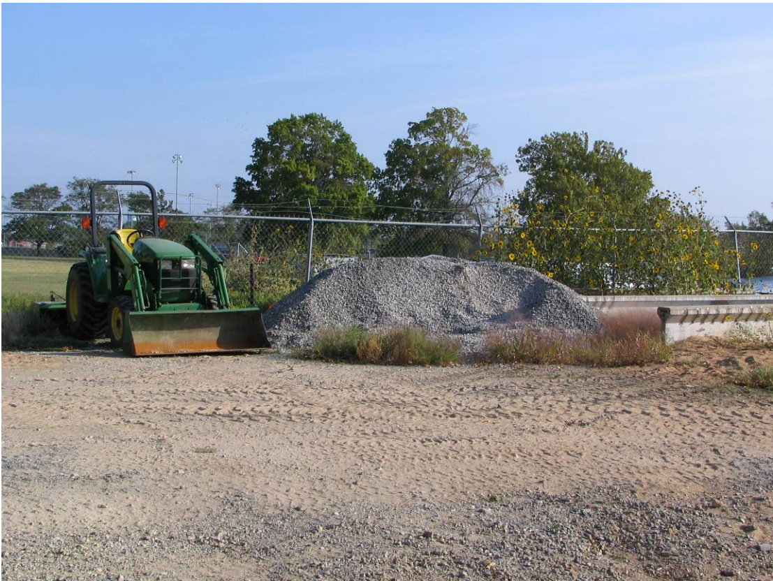
Figure 26: Coarse aggregate pile
