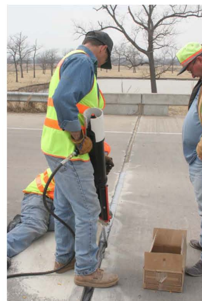
JOINT SAW AND SEAL
