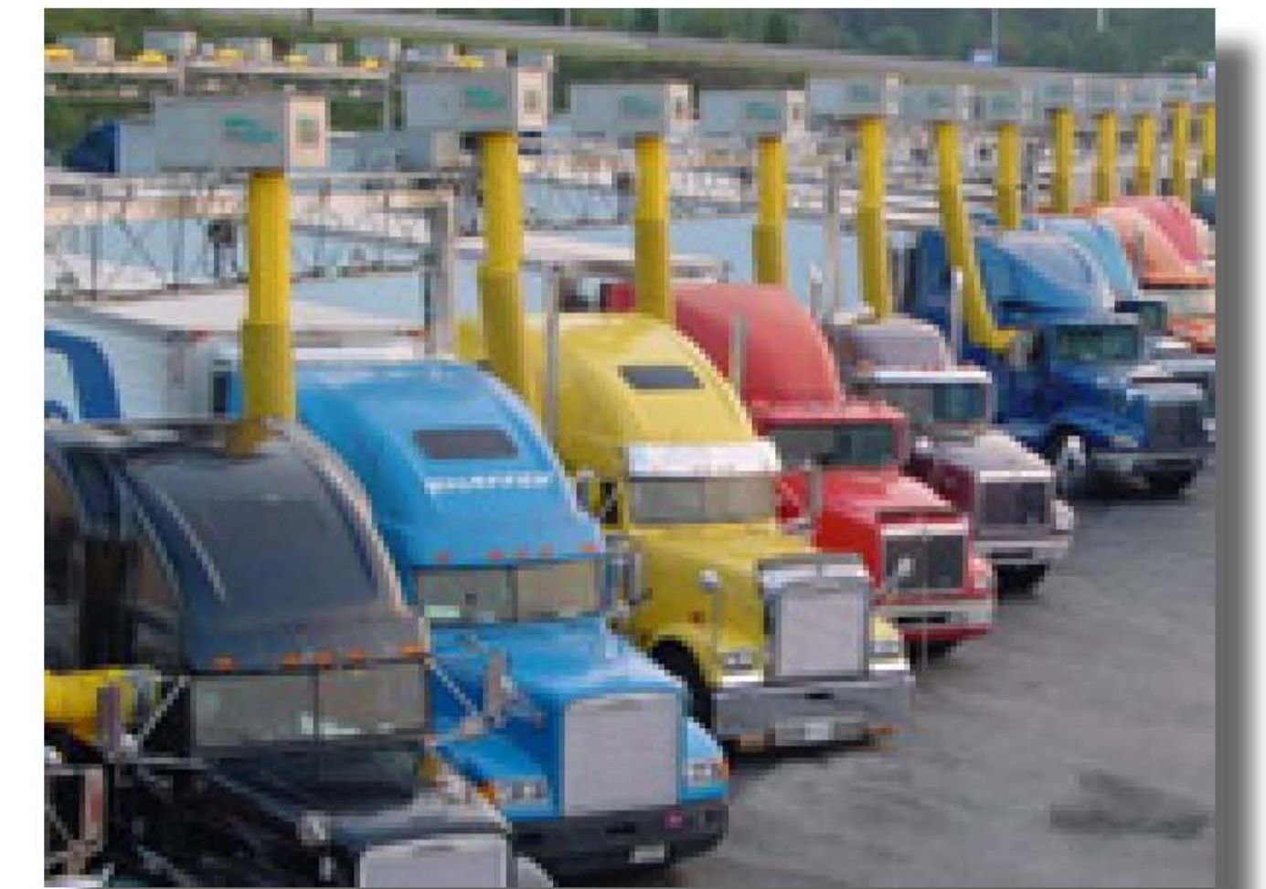
TRUCK STOP ELECTRIFICATION
