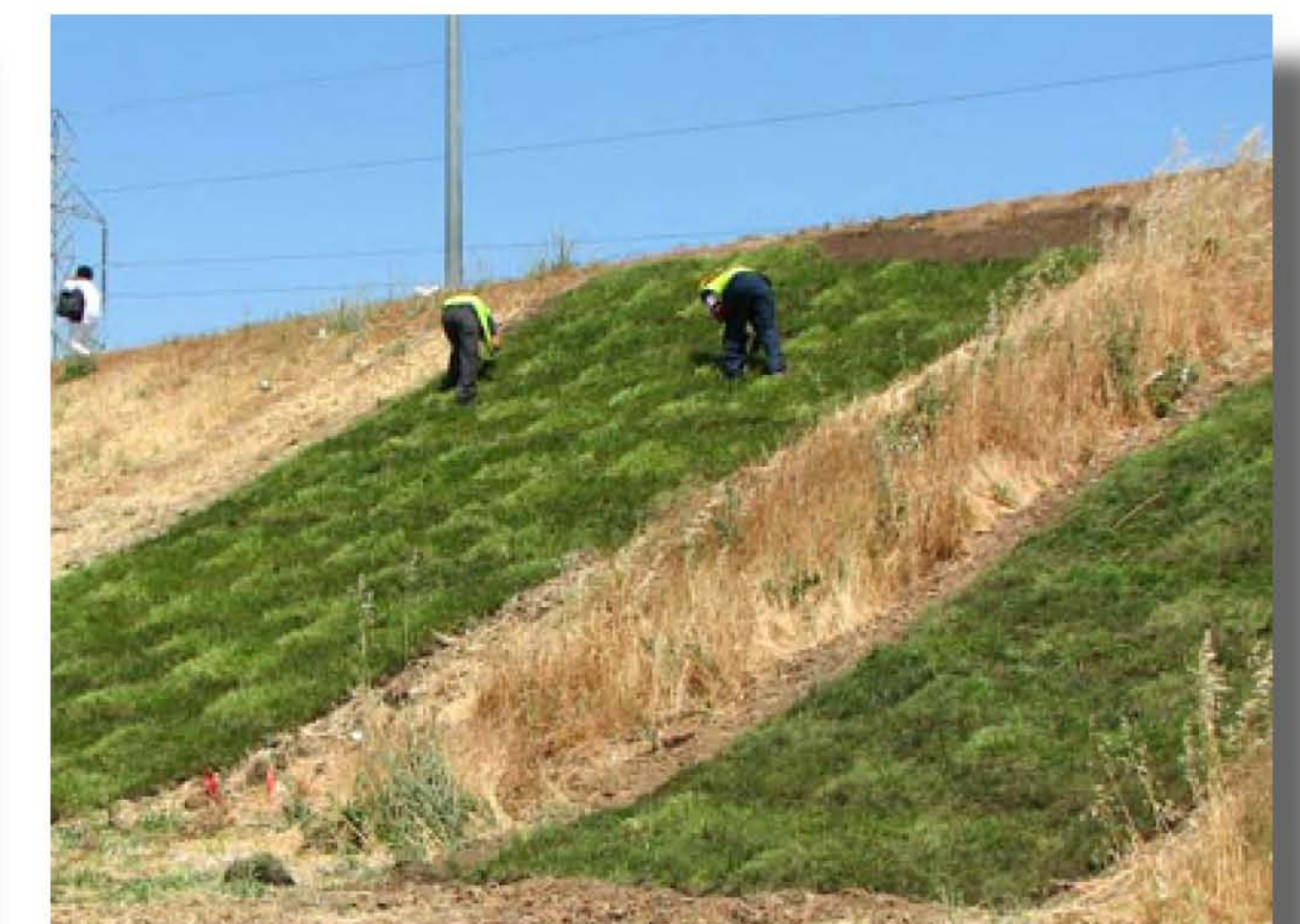
SOD EROSION CONTROL
